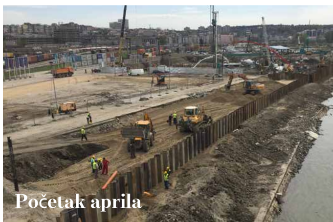
Gradilište BW Residences
